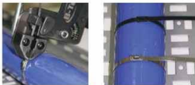
Application of Roller Ball Lock Ties
